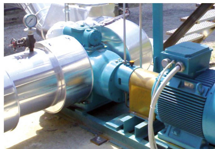
Pump solution for circulation of viscous products (asphalt, bitumen) in storage tank to ensure homogeneous product quality at all tank levels.
